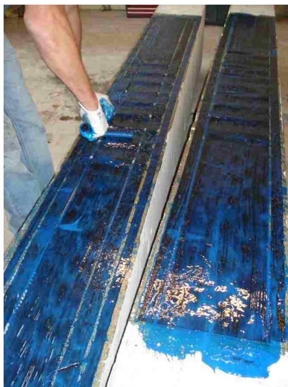
Figure 4.29. Ensuring Proper Bonding
