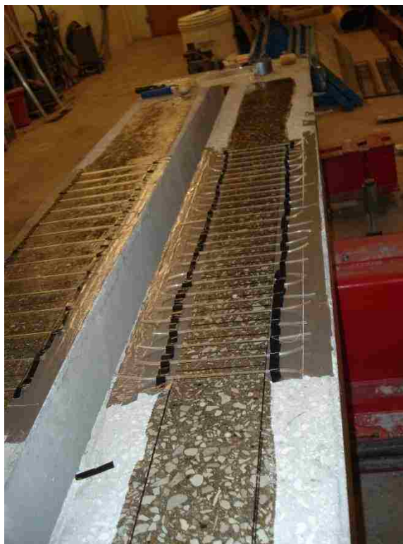
Figure 4.8. During FRP Application
